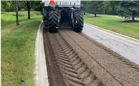
Grind existing pavement and gravel base into a new uniform base material. Grade and compact, then pave new layer of asphalt.
